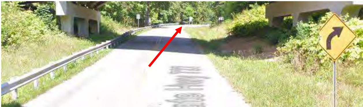
PHOTO 5: 5 TH STREET ROAD (EB) AT SCUFFLETOWN RD
