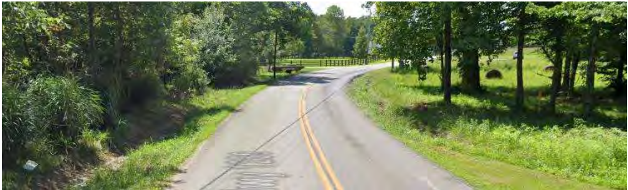
PHOTO 4: 5 TH STREET ROAD (WB) WEST OF I-75
