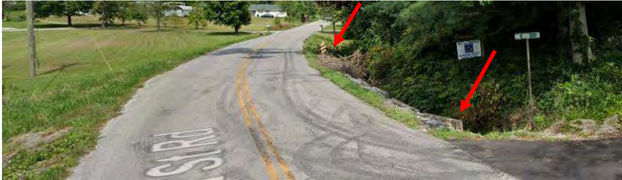
PHOTO 3: 5 TH STREET ROAD (EB) AT PINEWOOD DRIVE
