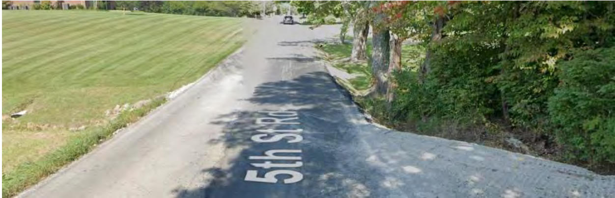
PHOTO 7: 5 TH STREET ROAD (EB)
