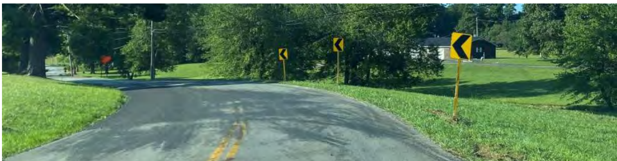
PHOTO 2: SB APPROACH NEAR ALSIP TRAIL
