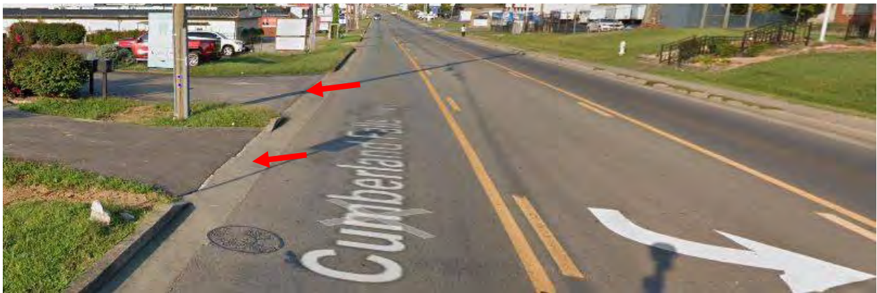
PHOTO 3: CLOSELY SPACED DRIVEWAYS (170 FT WEST OF 7 TH STREET RD)
