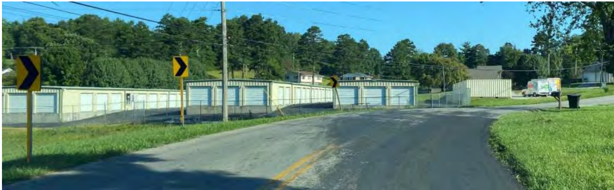
PHOTO 1: NB APPROACH NEAR ALSIP TRAIL
